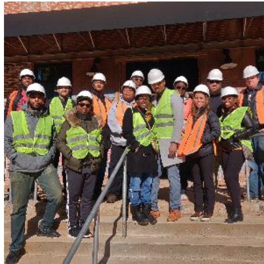
Another chilly but successful Thursday morning hard hat tour of Pittsburgh Yards and The Nia Building. The tours are held every Thursday at 10:45 a.m.
